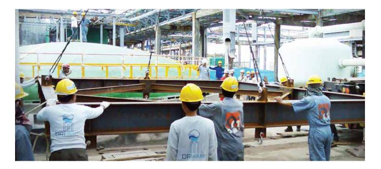
We are able to manufacture our tanks at your site/ project area (up to 3,000 cubic meter and with a height of up to 16,000 mm)
